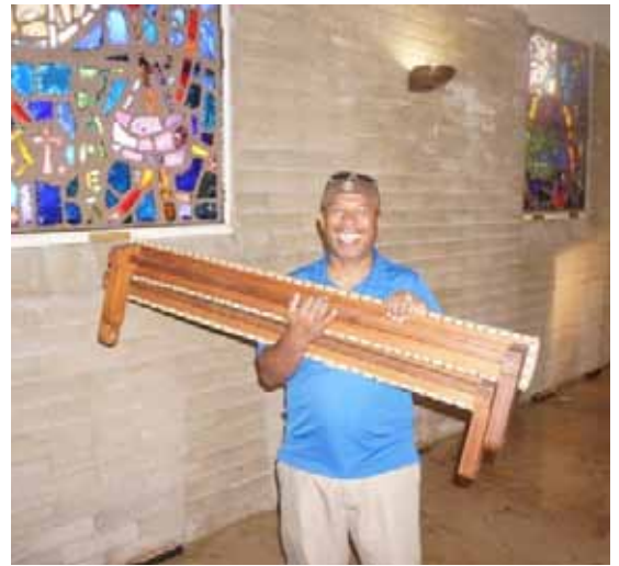
Marsono Remigio hard at work in the chapel restoration.
